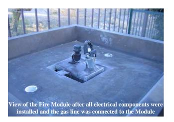
Once all the components were installed and the gas line was attached to the inlet side of the Fire Module we created a support bracket that we attached to the Fire Module. As seen in the photo at left, the support bracket held the Fire Module suspended in the hole in the top of the Small Pyramid.
