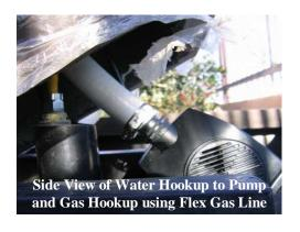
Once we had our flexible hose attached to the plumbing inside the Large Pyramid the next step was to connect the water pump which comes with this kit and extend the gas and electric up through Large Pyramid.
