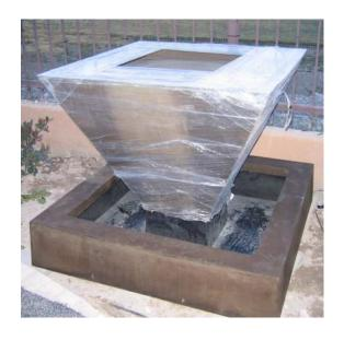
The photo at left shows the Large Pyramid after we installed the flexible water line to the plumbing inside and set it on the hard plastic base.
