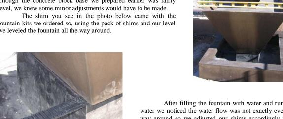
After filling the fountain with water and running the water we noticed the water flow was not exactly even all the way around so we adjusted our shims accordingly until the water flow was even. Afterward we trimmed our shims so they would not be visible. Trimming these plastic shims is just a matter of snapping them off as close to the base as possible.
